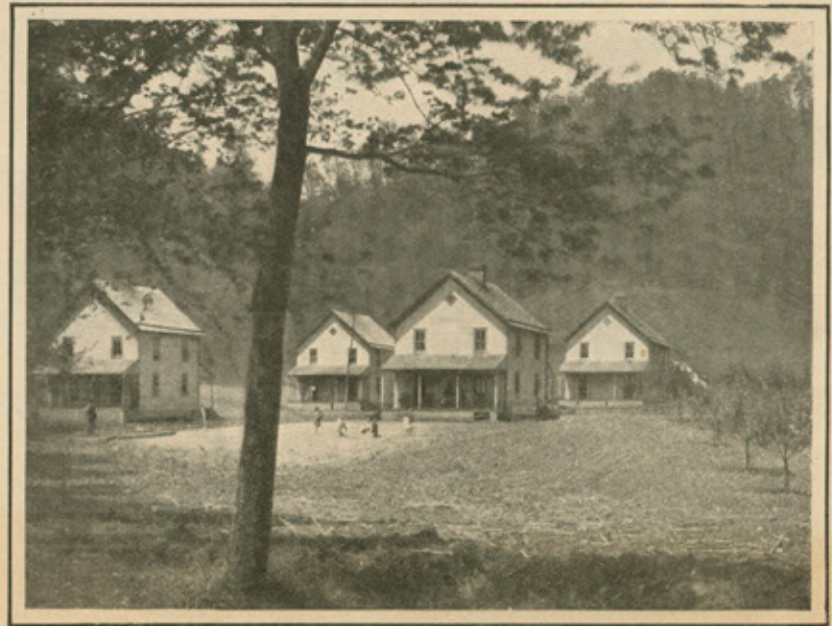
These are some of the cottages which have been erected by the students in order to pay their room-rent
