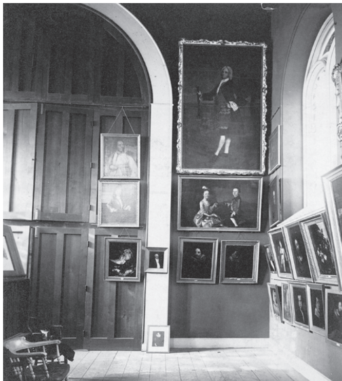
Banister Hall, second floor gallery, currently the Austin Organ windchest and pipes. Courtesy Bowdoin College Archives (#1360).
